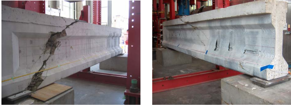
Fig. 6 Ultimate failure of girders AASHTO2C (left) and AASHTO2R (right)
