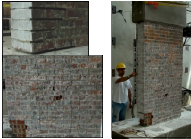
Fig. 4: Failure of the wall after first testing (cracking and crushing of bricks and mortar joints)
