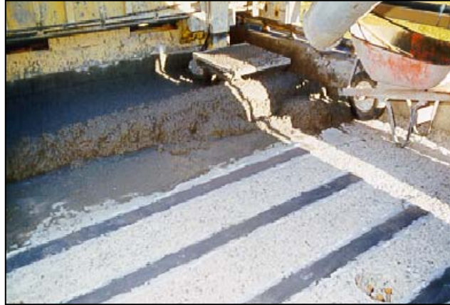
Fig 3: Placing CFRP Strips on Deck Slab
