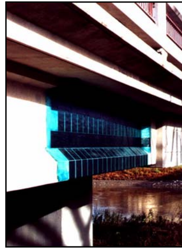
Fig. 5 (b) – Shear Strengthening of the Maryland Bridge
