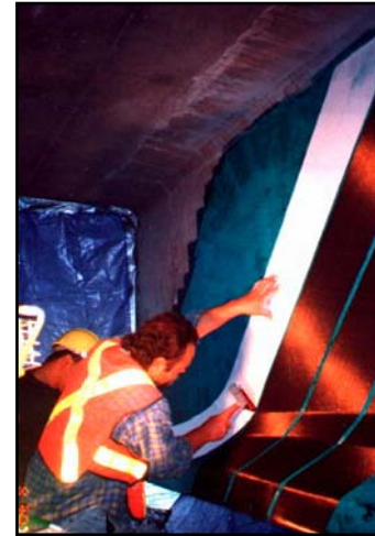
Fig. 4 (a): John Hart Bridge, Prince George BC Fig. 4(b): CFRP Application
