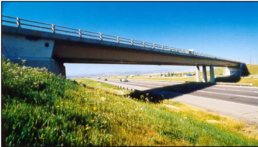
Fig. 1: Country Hills Boulevard Bridge over the Deerfoot Trail
