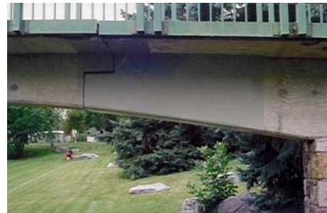
Fig. 8 (a): Application of CFRP Sheets Fig. 8 (b): Bridge After Repair
