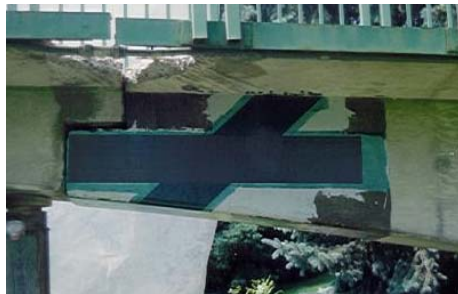
Fig. 8 (a): Application of CFRP Sheets Fig. 8 (b): Bridge After Repair
