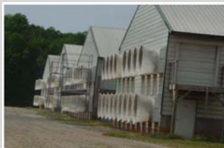
Three ventilated barns with 17-40' fans or both ends of each barn
